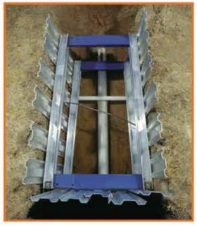
Waler with hydraulic struts is designed to allow 3- or 4-sided protection.
